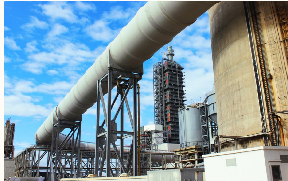
A fiberglass duct routes the flue gas from the generating unit to the carbon capture system at Petra Nova. Photography courtesy of NRG.
