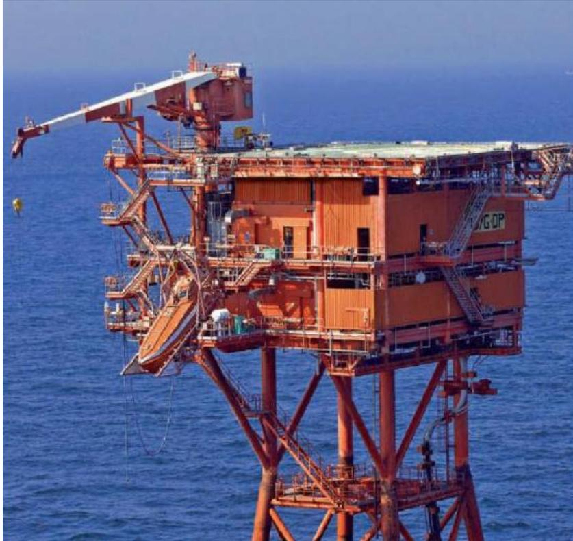
The topside consists of a Helideck, Mezzanine deck, Production deck and Subcellar deck and facilitates six wells. The distance between the deck legs is 10.000 [m] x 10.000 [m]. The jacket structure comprises of four tubular jacket legs braced by horizontal framings at EL (+) 6.000 [m] and EL (-) 25.000 [m]. The platform is founded on four piles of 1070 [mm] outside diameter and 40 [mm] wall thickness. These piles are driven through the legs and are welded on the top.
