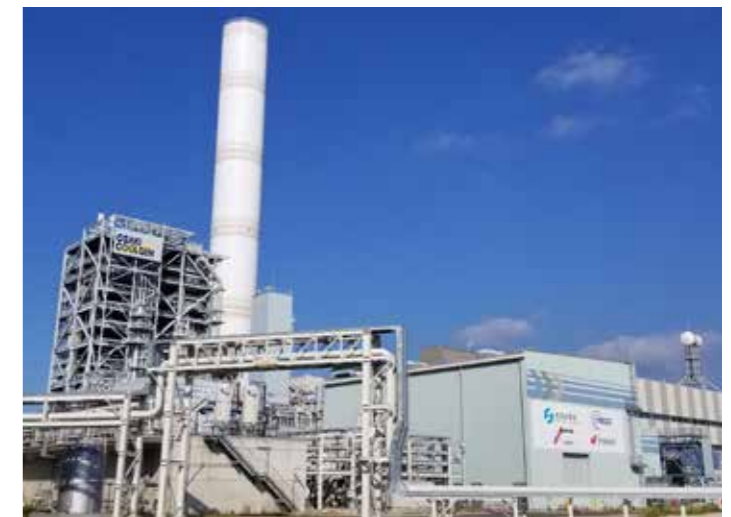
Osaki CoolGen facility, Japan.
