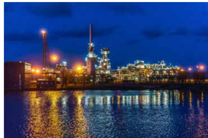
St Fergus Terminal, United Kingdom. Photo credit: North Sea Midstream Partners (NSMP).
