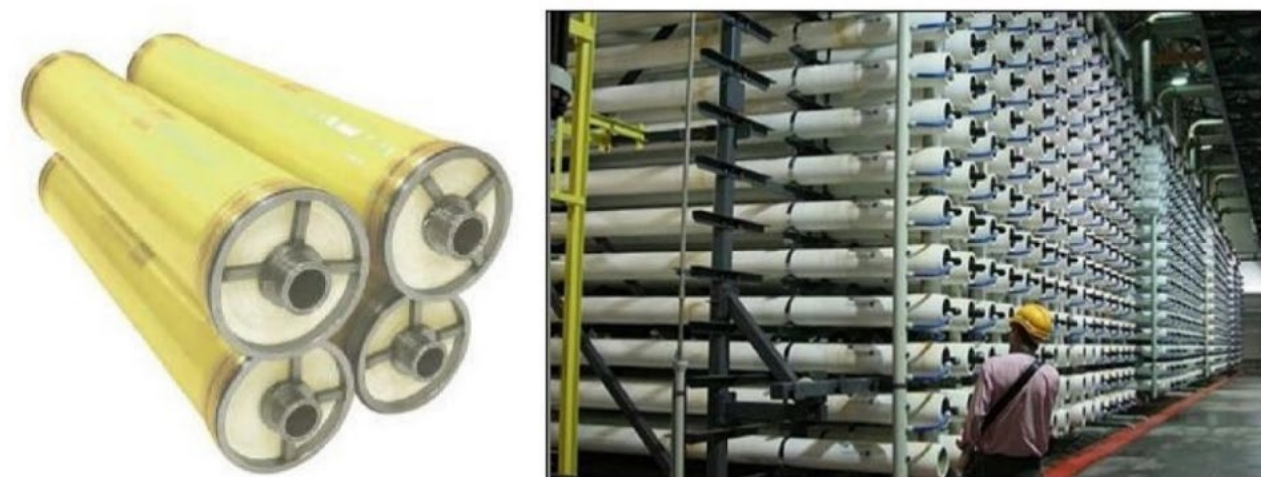
Figure 6 - Photos of spiral-wound membrane vessels (left) used in a commercial scale membrane system (right). Source: (NETL 2018).
