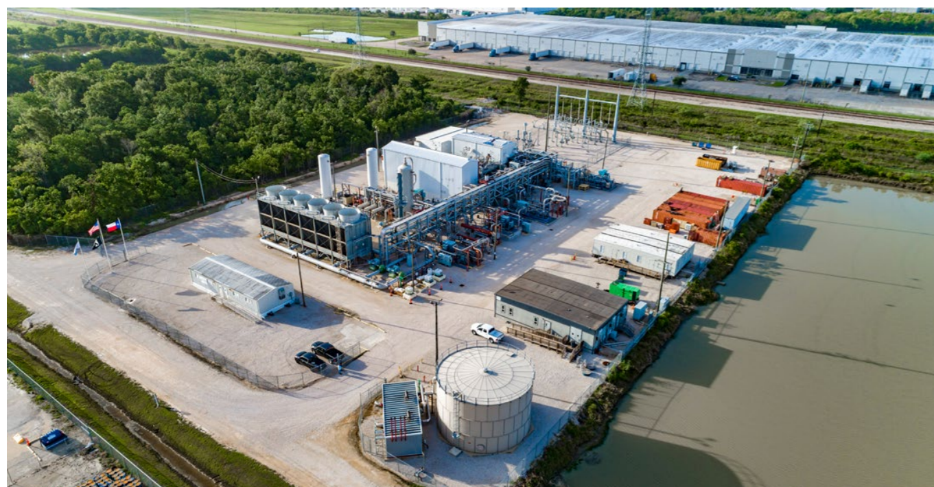
Figure 2: NET Power's La Porte Demonstration Facility
