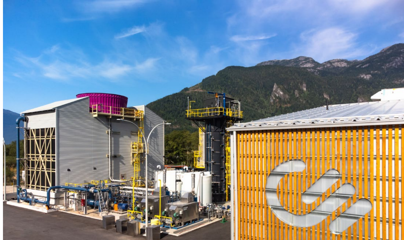
Carbon Engineering's Innovation Centre and Research & Development Headquarters located in Squamish, Canada.
