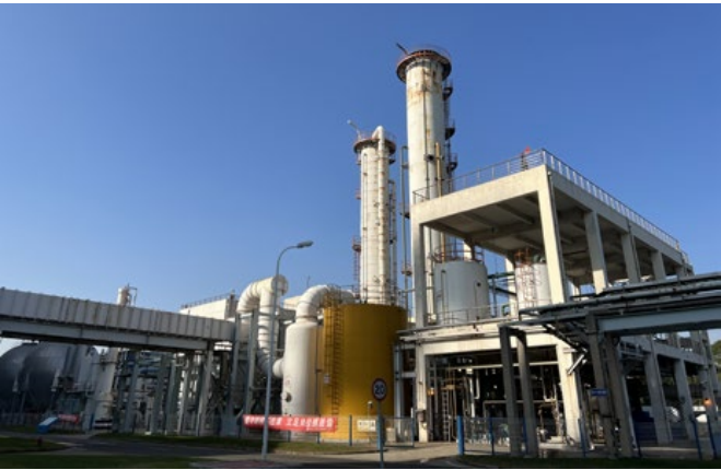
1. Shanghai Shidongkou 120,000 tonne/annum phase-change CO 2 capture project.
