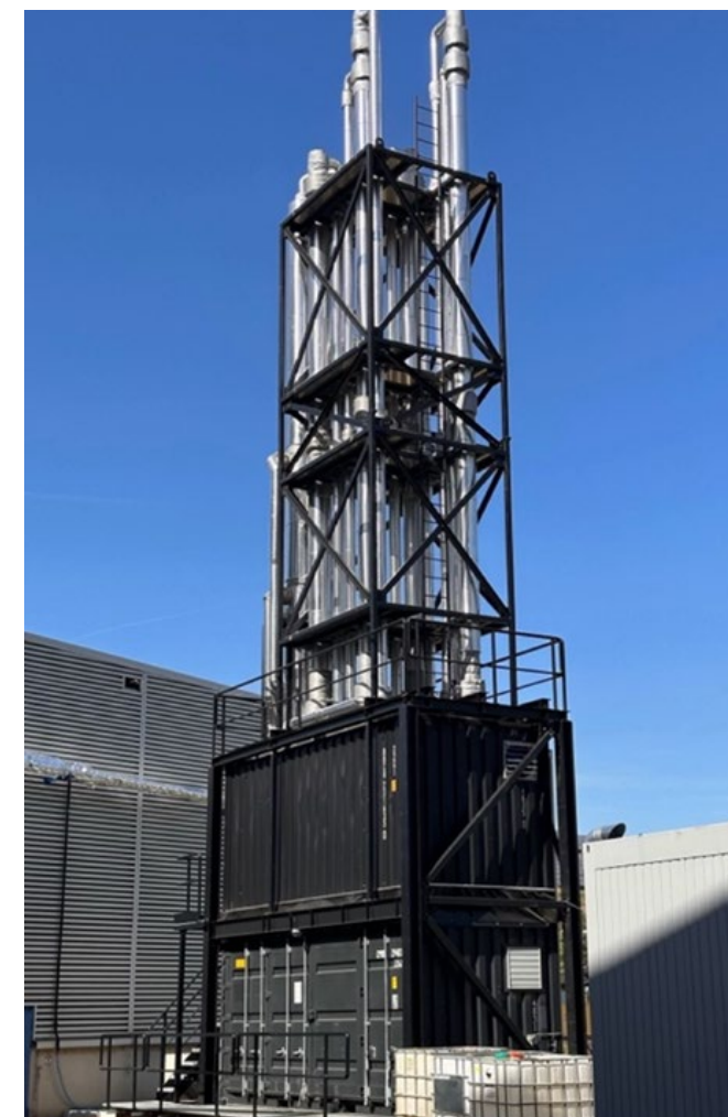
CapsolGo® unit 2 at German EfW (Energy-from-Waste) plant.
