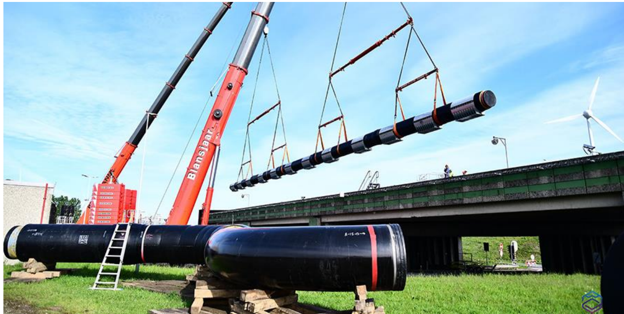
CO 2 pipeline being installed in Rotterdam, Netherlands Source: Porthos Project
