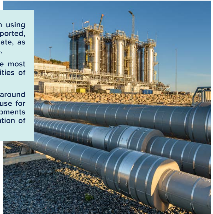
Northern Lights onshore pipeline, Norway. Image courtesy Northern Lights JV
