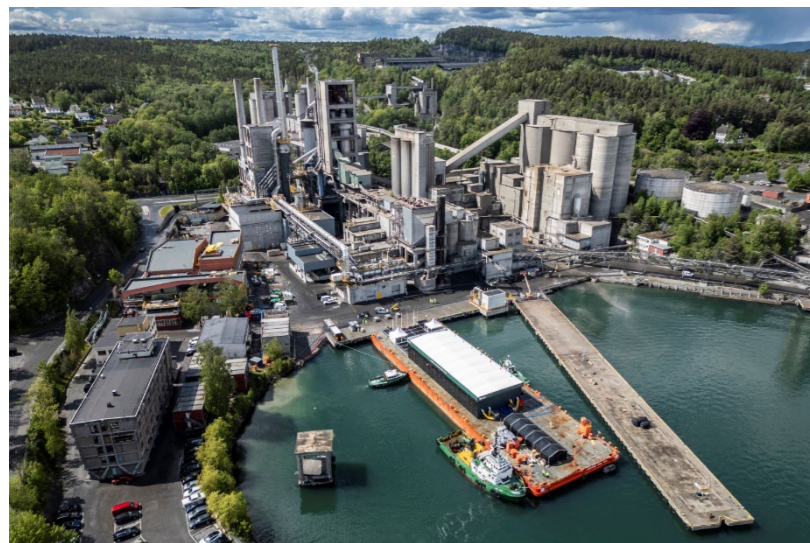
Brevik CCS Facility, Norway, image courtesy SLB Capturi and Heidelberg Materials
