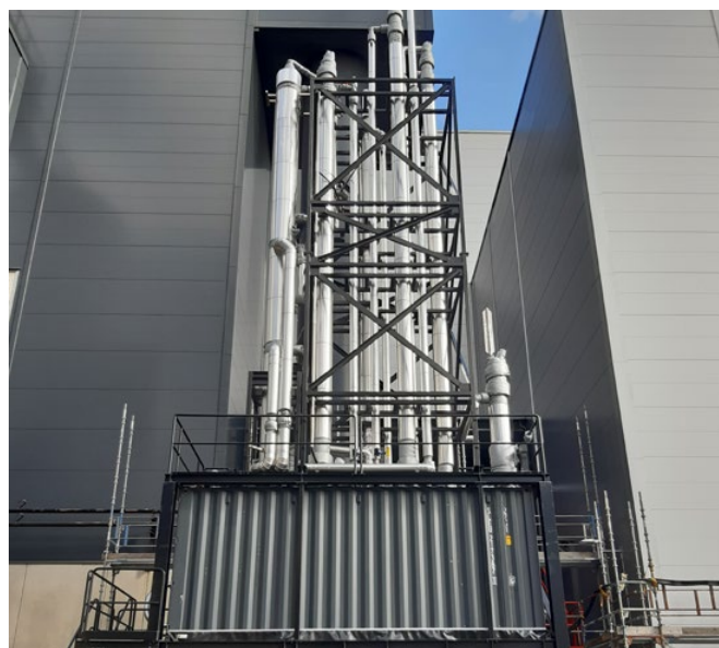
Sumitomo SHI FW (SFW), together with partner Capsol Technologies ASA, and Swedish energy company Vaxjö Energi AB collaborated on a testing campaign to demonstrate carbon capture technology based on the Hot Potassium Carbonate (HPC) process.
