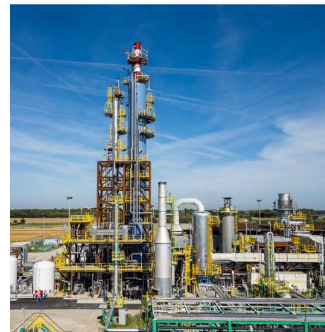
NX DECARB™ industrial application - Energy integrated post combustion carbon capture at the Casal Borsetti site (Italy) (image courtesy of ENI)
