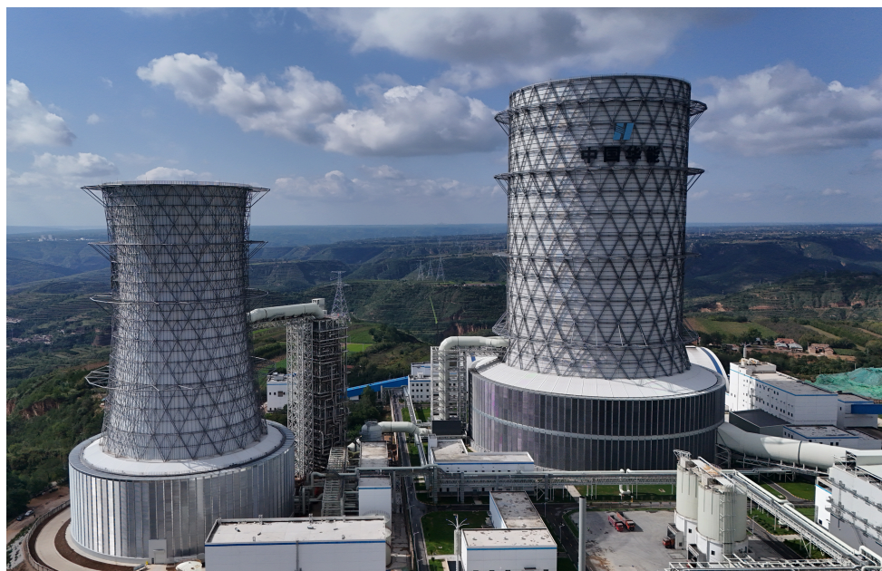
Longdong CCS Facility
