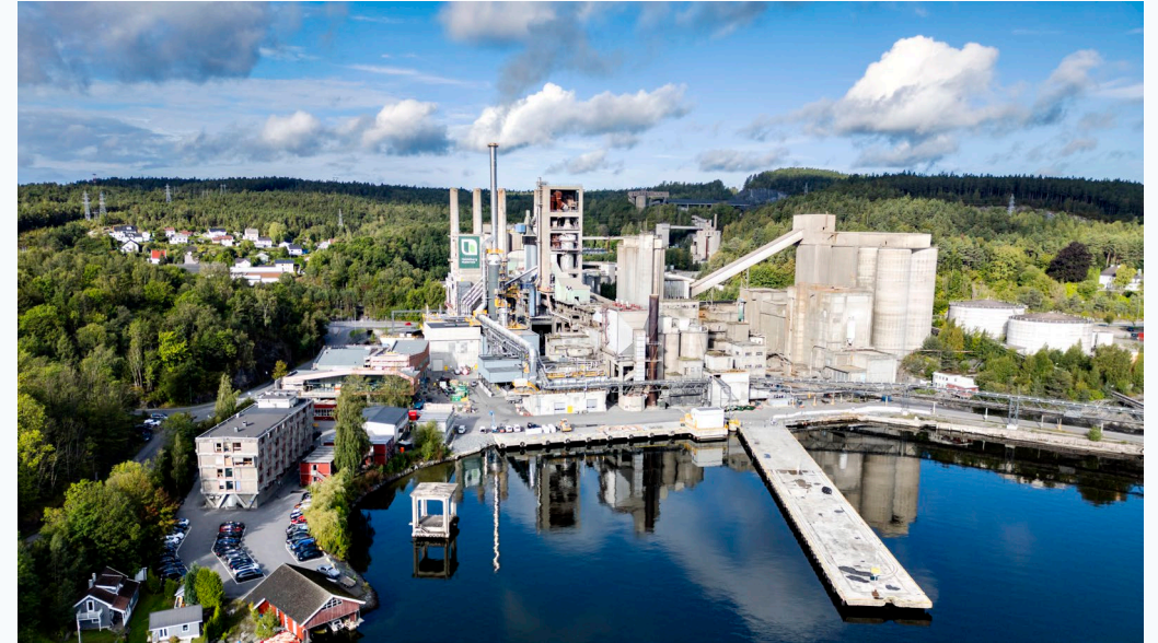
The Brevik CCS facility in Brevik, Norway. Image courtesy carbon capture technology provider SLB Capturi.
